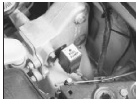
2.3c On 1992 models, the fuel pump relay is located in the left rear corner of the engine compartment
