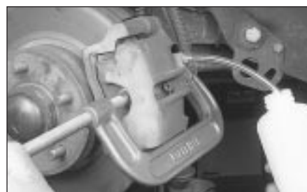
3.5b Attach a hose to the bleed screw, open the bleed screw slightly and depress the piston into the caliper. Tighten the bleed screw when the piston bottoms
