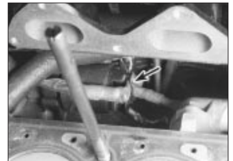
15.4b From underneath the vehicle, remove the cylinder terminal from the solenoid (cylinder head removed for clarity)
