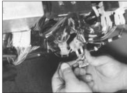
6.9 Check for battery voltage to the IGN ON relay
